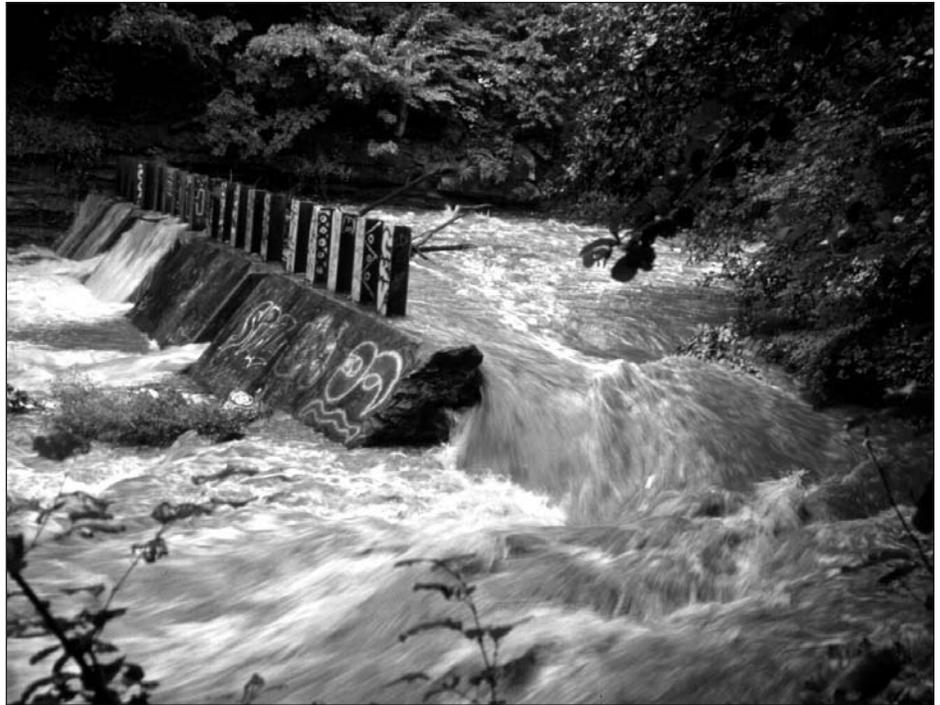
**Figure 7-4** Erosion around the end of the trash rack upstream from Martin Luther King, Jr., Boulevard is one result of high flows in Doan Brook. Photograph by L. C. Gooch
